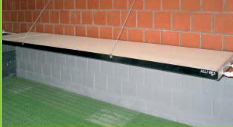
Radiated heat can only be felt as heat when it strikes an object and is therefore not affected by ventilation or draughts. Convected heat, on the other hand, heats the air directly under the panel so that the piglets are attracted to the warmer climate under the panel.
